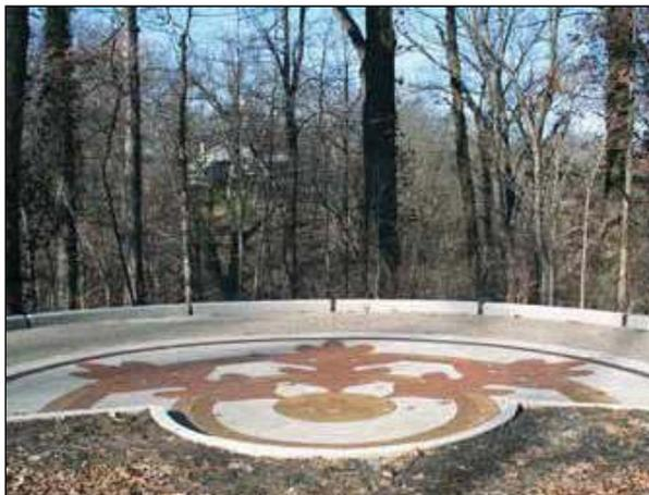
The 4,120-square-foot area was constructed using eight inches of pervious concrete paved over a 12-inch base of clean No. 57 gravel.
