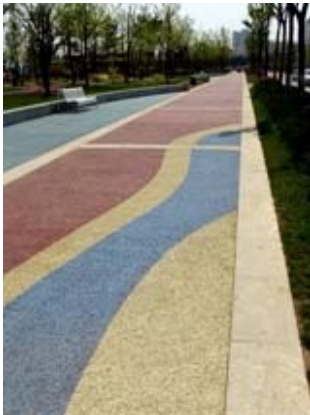
Large expanses of colored pervious concrete are being installed at Olympic venues in and around Beijing. When liquid pigments are used, the water content of the mix must be adjusted to account for liquid in the pigments, keeping the w/c ratio accurate. Photo: Bunyan Industries, USA
