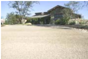
Black Mountain Ranch House is the 28th building in the world to obtain Platinum LEED status, an achievement due in part to the pervious parking area, driveway, and walkways. Photo: Davis Colors
