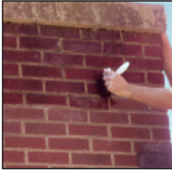
Apply DRYLOK® 5% SILICONE generously with a brush.
