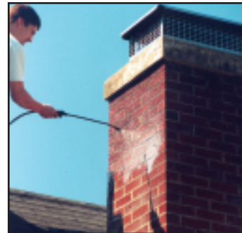
Apply DRYLOK® 5% SILICONE by flooding the surface with a garden sprayer.
