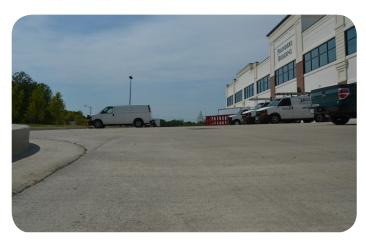
Not only does it save money, but less finishing of the concrete, including the elimination of troweling, actually improves the quality and durability of the concrete.
