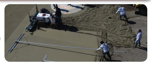
The placement was done with a Somero S-840 ride-on laser screed. This dramatically decreased construction time. The finishing was quick and simple. After screeding, all that was involved was an initial bull float, a medium broom finish, a cure and seal application and then the joints where saw cut.
