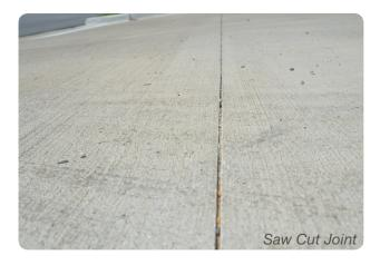
There are three types of joints: *Contraction Joints, Construction Joints and Isolation joints.*
